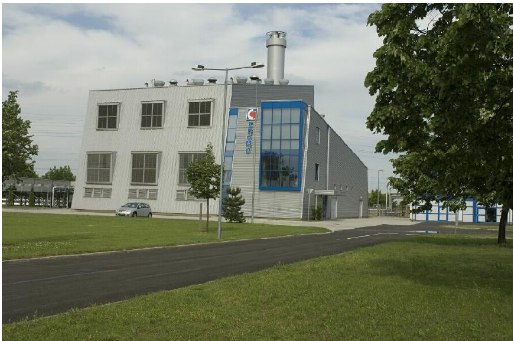
Picture 2 Wärtsilä 18V34SG gas CHP application (12 MW) in Győr, Hungary
