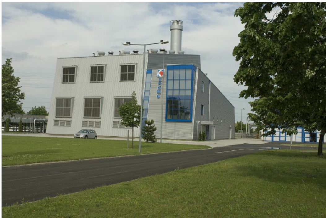
Picture 2 Wärtsilä 18V34SG gas CHP application (12 MW) in Györhö, Hungary
